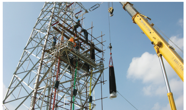
Submarine cable accessories installation
