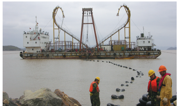
Daishan-Dajiaoashan submarine cable installation
